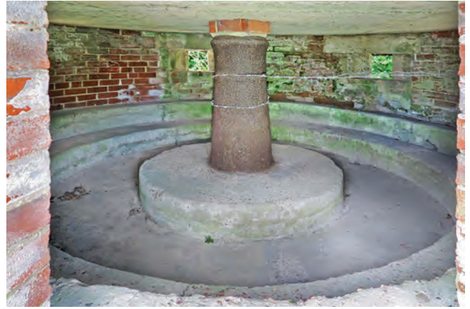
Improvised twice, a WWI AA gun mount made of an old cannon later enclosed as a WWII pill box. Photo Clive Penfold
